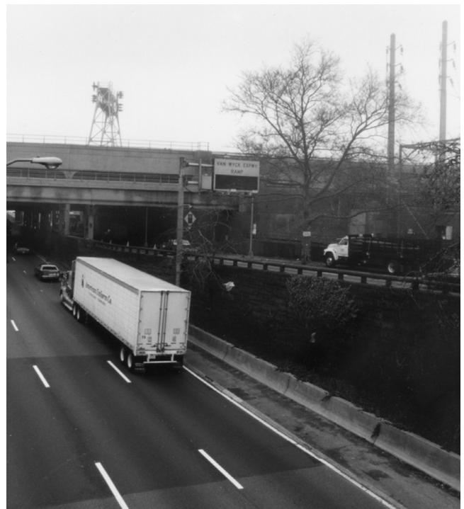
FIGURE A.3.3.23.1 Depressed highway.
